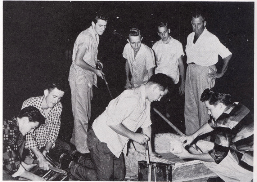
J. R. Daniel watches as members of the Glo-Blok Company mix concrete.
